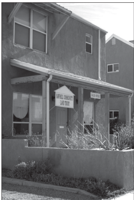
Above and opposite: a large-scale inner-city redevelopment project completed by the Sawmill Community Land Trust in Albuquerque, New Mexico, USA.
